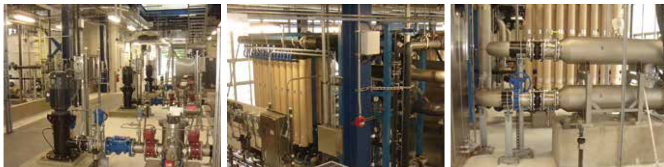
▲ Figure 1. The Univ. of Connecticut Storrs campus installed a two-stage reverse osmosis system with microfiltration pretreatment to treat reclaimed water for use as boiler makeup. Shown here (left to right) are some of the components that pretreat the water prior to RO: the pump that feeds water to the microfilter system, the microfilter membrane cartridges, and the UV reactors. Photos courtesy of Jason Maskaly.
