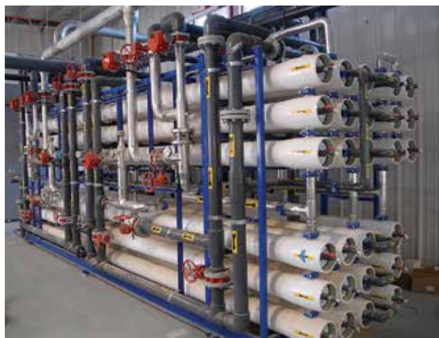
▲ Figure 4. This low-pressure reverse osmosis (LPRO) system can provide up to 650,000 gpd of reclaimed water to a snack foods plant.
