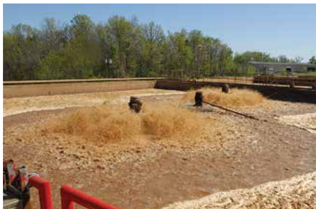
▲ Figure 2. This activated sludge aeration tank at a pork processing plant is equipped with floating mechanical aerators.
